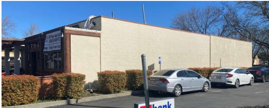
Side (south) façade, view facing northeast. Source: ESA, 2024.
