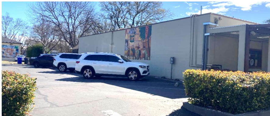
Side (north) façade, view facing southeast. Source: ESA, 2024.
