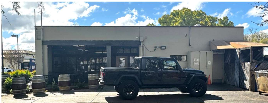
Rear (east) façade, view facing west. Source: ESA, 2024.
